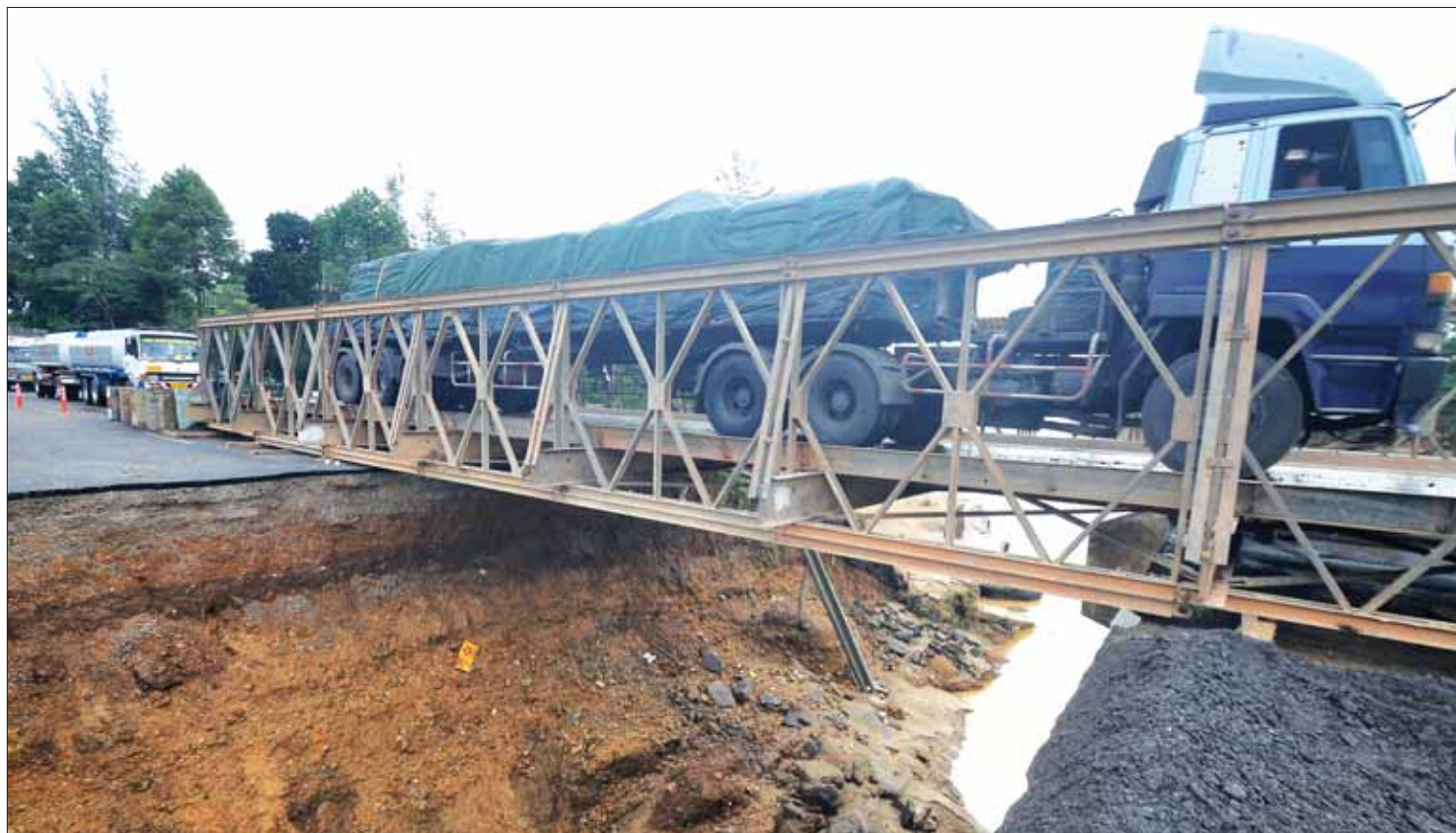
Vehicles cross over flood-damaged Wang Yao Bridge using a 'Bailey Bridge' that has been installed to resume traffic. Photo: The Nation
