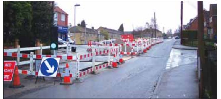
Even the smallest maintenance project on British roads features a plethora of safety signs, barriers, lights and reflective cones. Photo: David Anstiss
