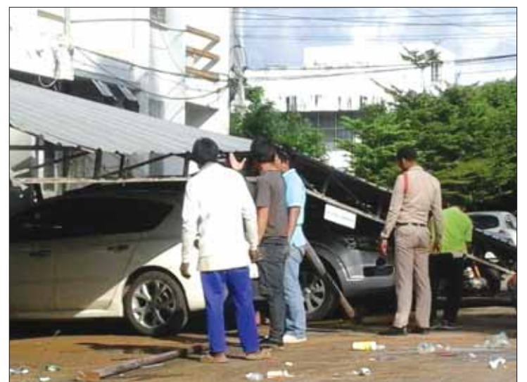
The crane driver claimed that he could not stop the crane, despite repeated attempts to brake. Photo: Kritsada Mueanhawong
