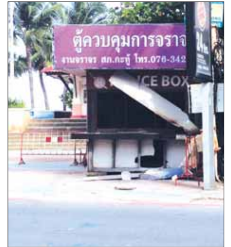
A device detonated at a police box at the end of Bangla Road in Patong. Photo: Patong DDPM
