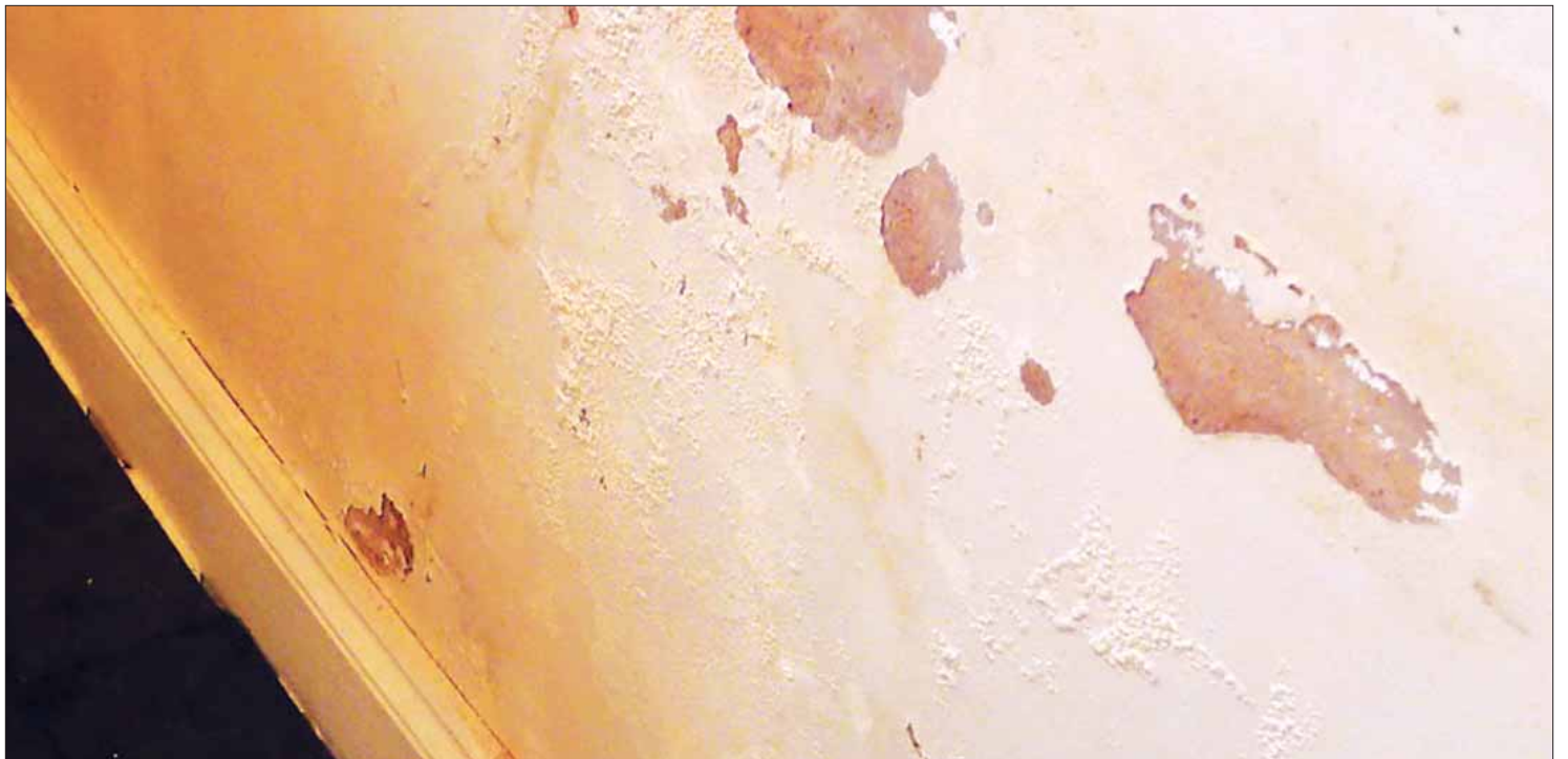
The temperature inside most homes in Phuket, in addition to surfaces that stay wet for extended periods of time is sufficient enough to support mold growth, be it on wood, paint, drywall paper or fabrics. Photo: Kebabknight
