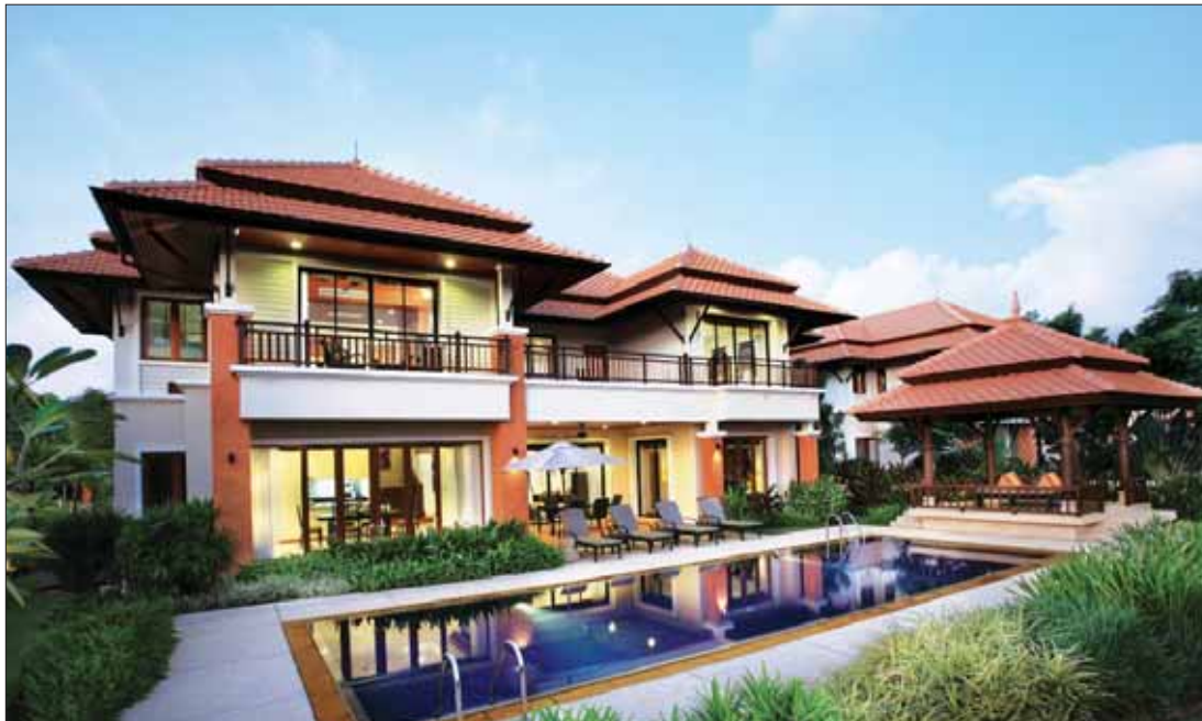
Four-bedroom villas (pictured above) are equipped with kitchenettes and balconies, are surrounded by gardens and have private swimming pools. Photo: Banyan Tree Hotels & Resort
