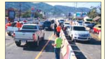
Samkong Underpass. Photo: Highways Department
