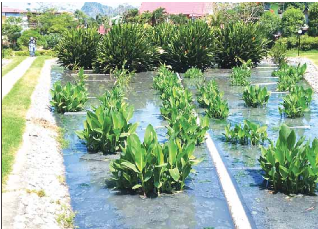
The Phi Phi treatment plant is not able to cope with the amount of wastewater produced. Photo: Gazette file
