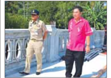
Gov Chamroen (left) inspects the flyover. Photo: Phuket PR
